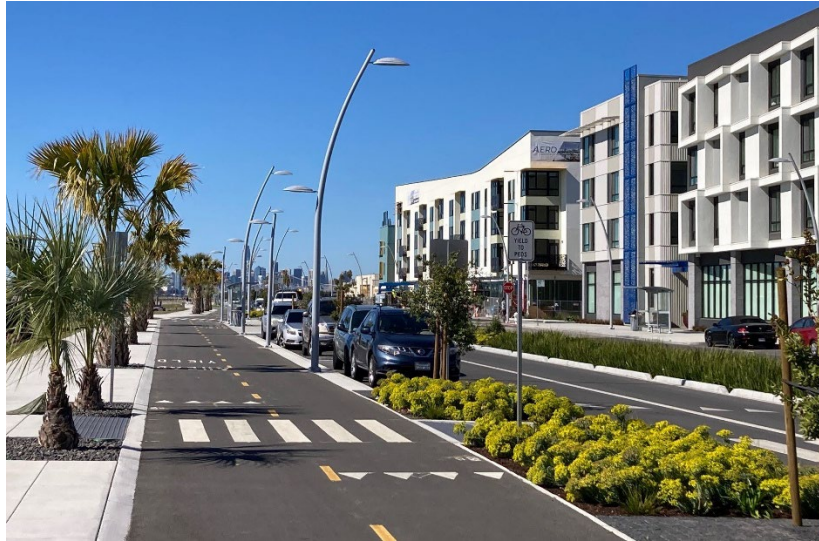
Cross Alameda Trail along West Atlantic Avenue
